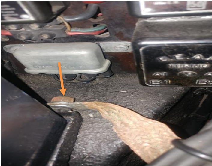
Copper ground strap going to engine block
